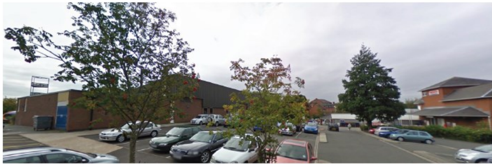
View 2 - Showing existing swimming pool viewed from the north
